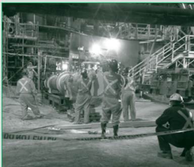
B&M crews prep saltwater piping at the Brunswick Smelter
