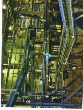
Conveyors Installed & Removed
