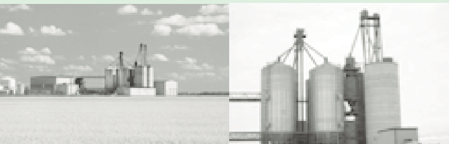
The APLP's Ste. Agathe, Manitoba facility, located just outside Winnipeg
