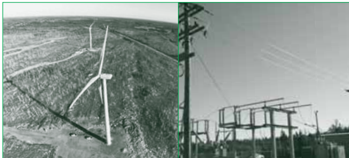
Atlantic Utility Region’s first major overhead line installation, and our first New Brunswick substation upgrade
